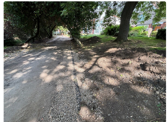
Flush drainage line along the tree-lined path
