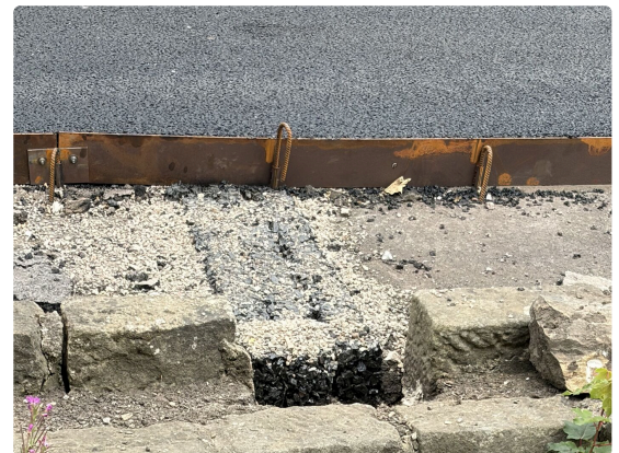
Grip Strip outlet through the heritage wall coping
